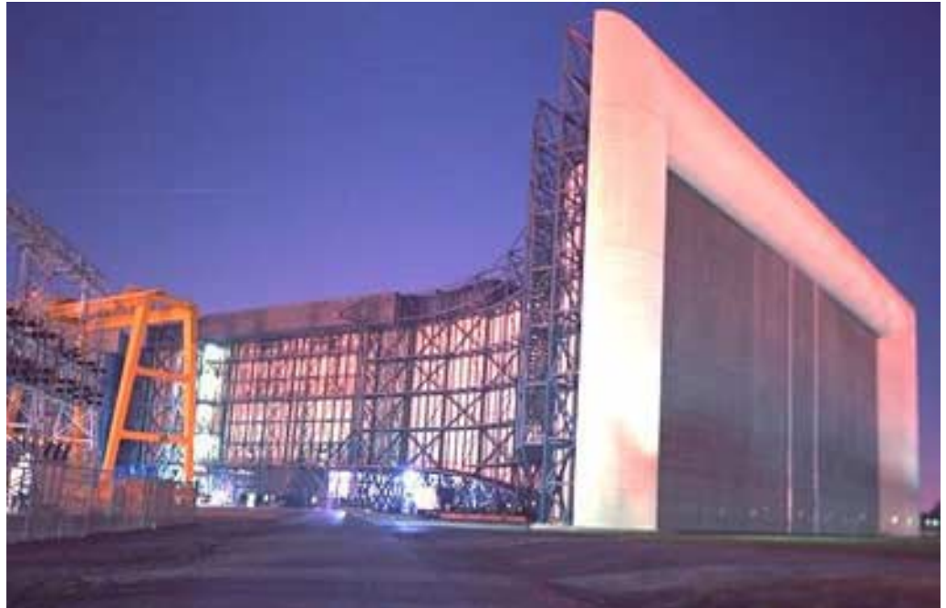
80x120 foot test section of National Full-Scale Aerodynamics Complex at NASA Ames.
